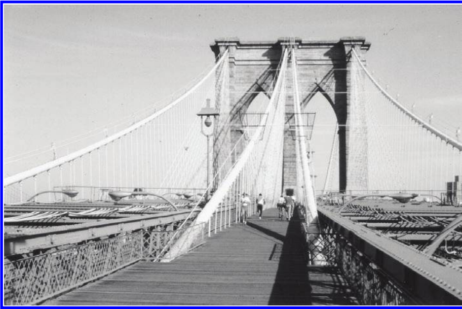
FIGURE 3.3 Brooklyn Bridge, New York. (Courtesy of Charles Seim.)
