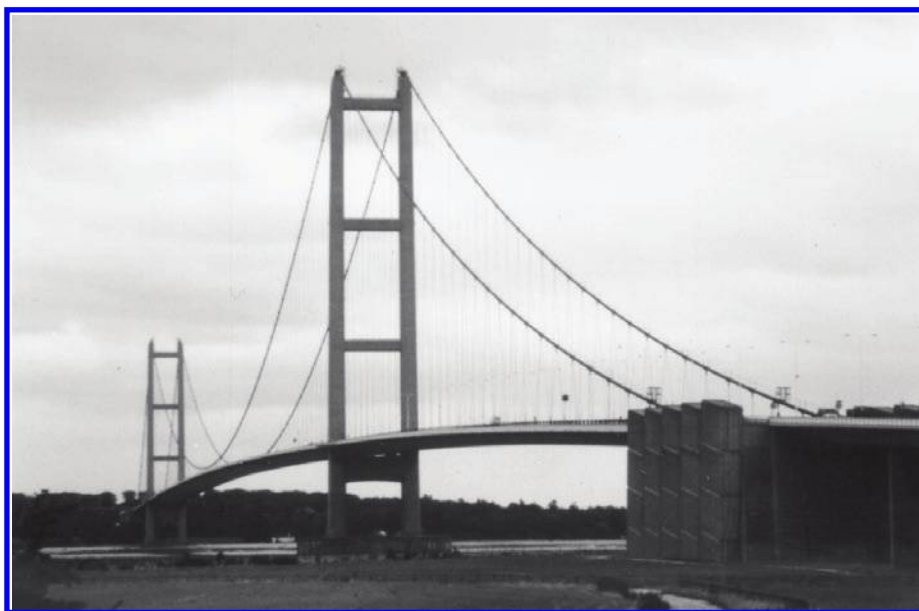
FIGURE 3.12 Humber Bridge, England. (Courtesy of Charles Seim.)
