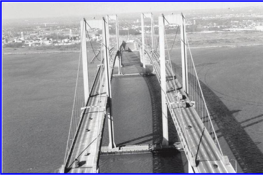
FIGURE 3.5 Delaware Memorial Bridges. (Courtesy of D. Sailors.)
