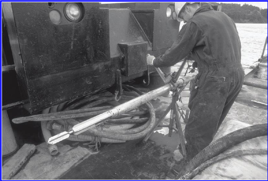
FIGURE 5.5 In situ vane shear device.
