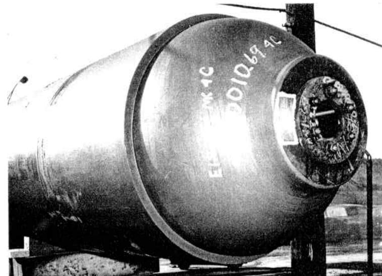
Fig. 7.28. Banded Vessel, Showing the Spherical Head and Banded Cylinder, being Installed at a Site
