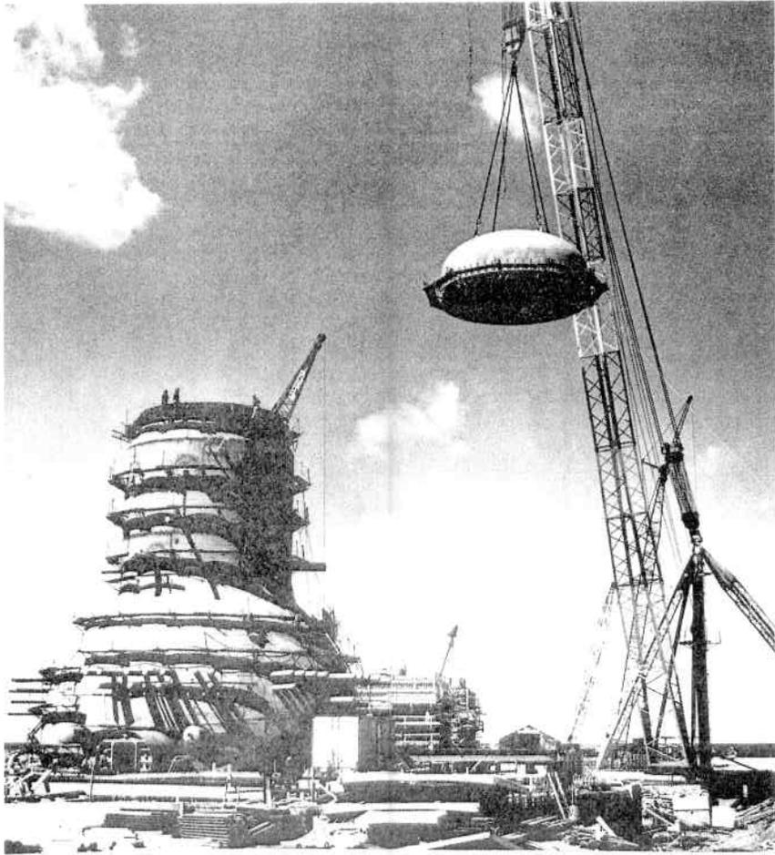
Fig. 2.1. Nuclear Power Plant Containment Vessel (Courtesy Chicago Bridge & Iron Co.)
