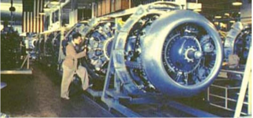
Aircraft engine is being assembled.
