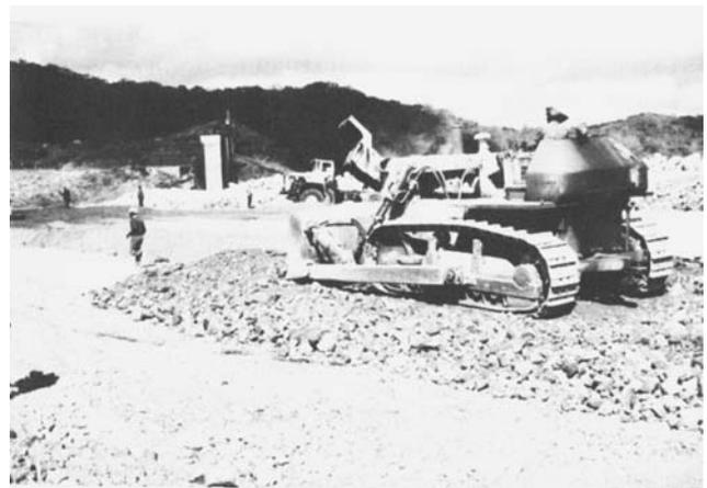
**Figure 59.8** Photograph showing segregation of crushed-rock transition materials at edge of windrow.
