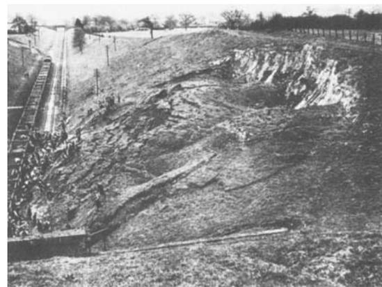
**Figure 47.7** Slide in very stiff fissured clay.
