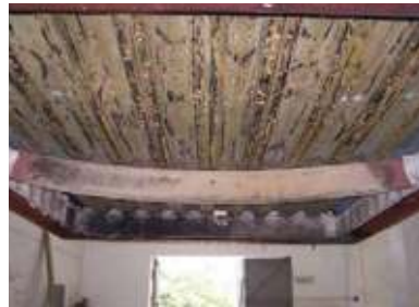
Fig. 9.24 Deformation at the bottom of S-2 after the test
