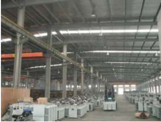
Fig. 11.1 Application of the steel portal frame
