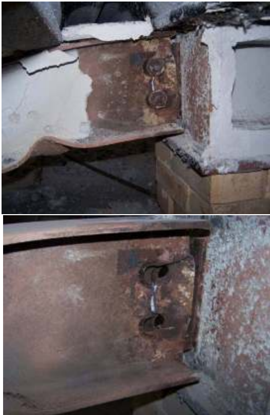
Fig. 7.40 Breaking of the joint in test CB150
