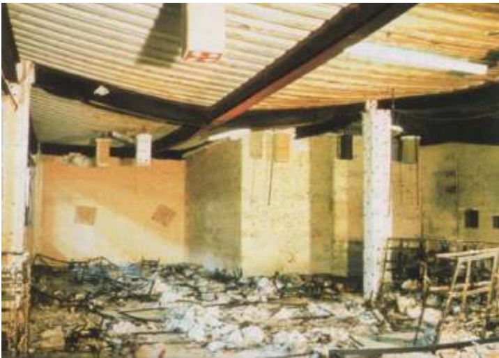
Fig. 9.10 Large deflections of the slab in the Cardington fire test
