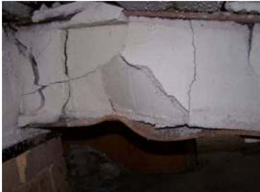
Fig. 7.41 Local buckling of the steel beam in test CB150
