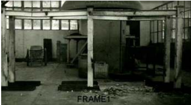
(a) Failure of FRAME 1
