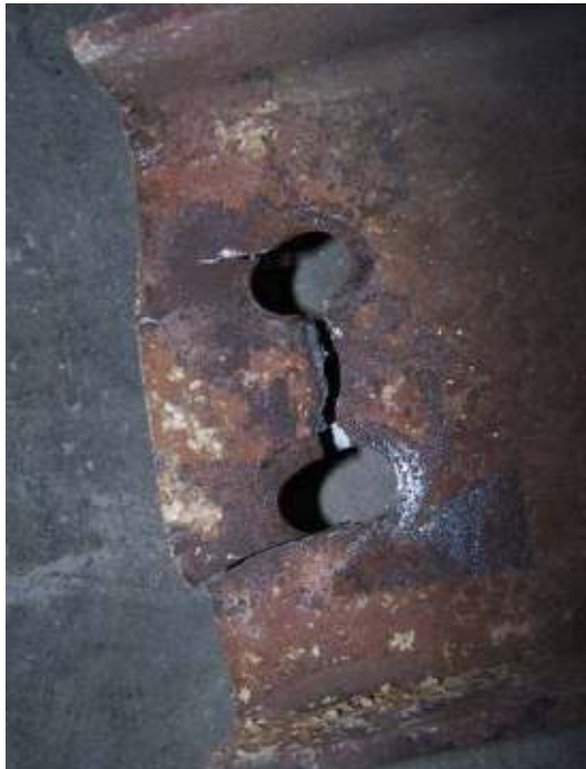
Fig. 7.42 Deformation of the web and high strength bolt in test CB150
