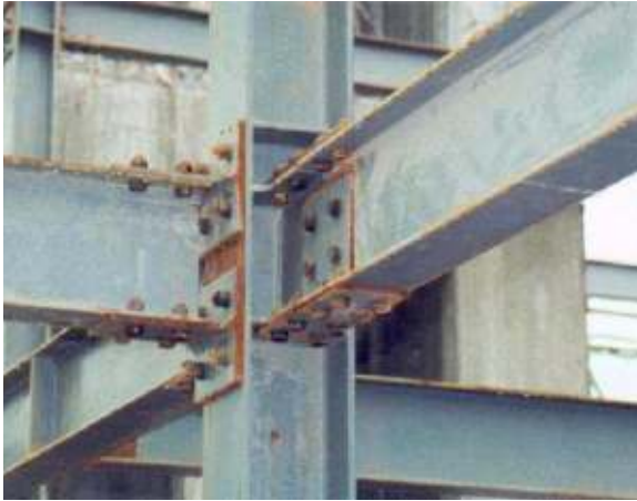
Fig. 8.1 Typical beam-column connection in a framed structure
