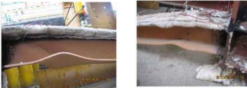
Fig. 7.8 Local buckling of the restrained beam
