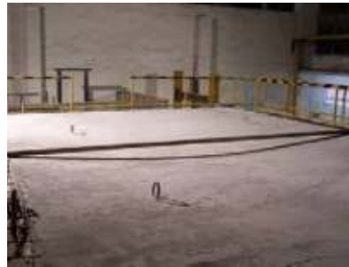
Fig. 9.22 Deformation of the slab after the test S-1
