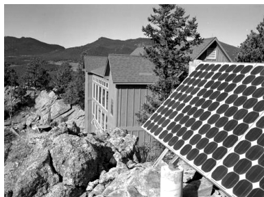
FIGURE 4.1 PV array located adjacent to residential building.
