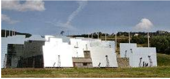
Fig. 11: The array of mirrors are controlled by a computer and turn with the sun.
