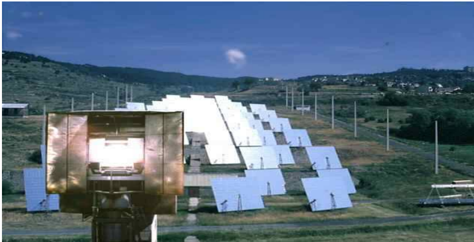
Fig. 19: The 63 mirrors (heliostats), each having an area of 45 \text{ m}^2 , with a combined area of 2835 \text{ m}^2 . The reflectivity is 0.79.
