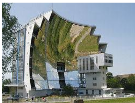
Fig. 10: The Solar Furnace of Odeillo; The parabolic shape of the giant solar collector is evident here.
