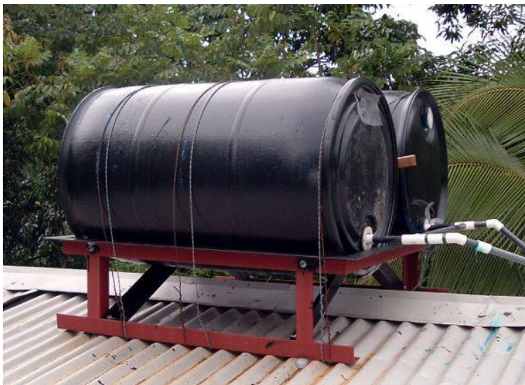
Fig. 54: A roof- mounted simple solar water heater.
