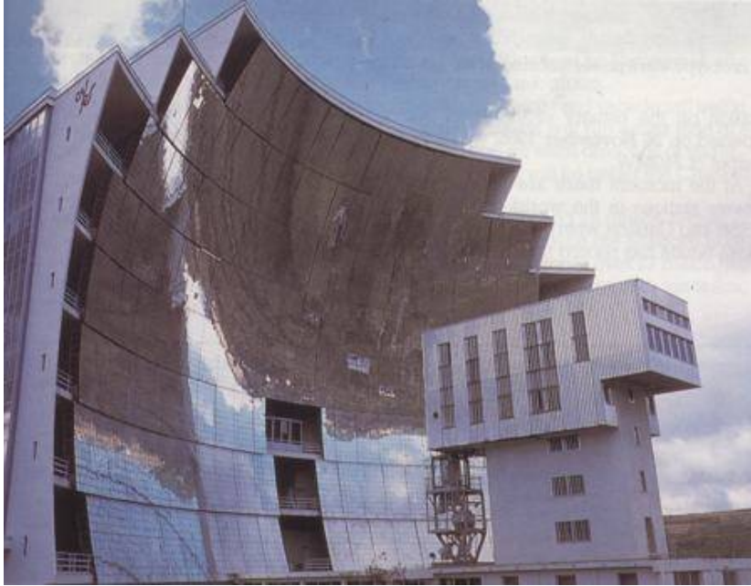
Fig. 21: A good view of the giant parabolic solar collector It has a reflective area of 1830 m 2 . The reflectivity is 0.79.
