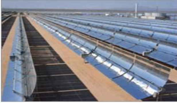
Fig. 52: For problems: The troughs are 100 long, 1m wide, and separated by 3 m. There are 100 troughs in the “solar field”.
