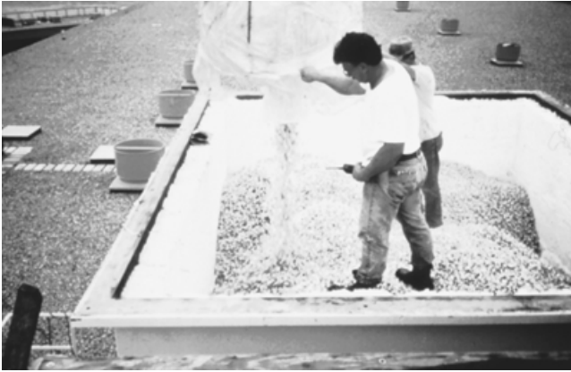
FIGURE 13.13 Loading random media. (Courtesy of Smith Environmental Corp.)
