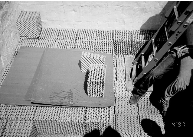
FIGURE 13.14 Installing structured media. (Courtesy of Geoenergy International Corp.)
